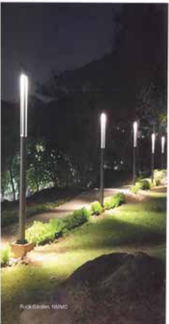
Riyadh Metro QCC Zone, Saudi Arabia
